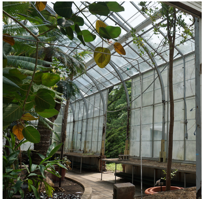
The hole created in the south wall of the Tropical House provided an exit for the larger trees.
